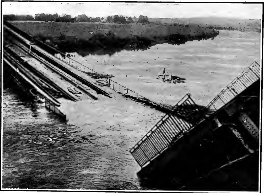
A BRIDGE OVER THE MEUSE. Destroyed by French Engineers.
